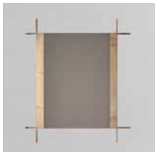
Cut a hole in the wall and install 2 wooden planks (dimensions: see technical data sheet)
